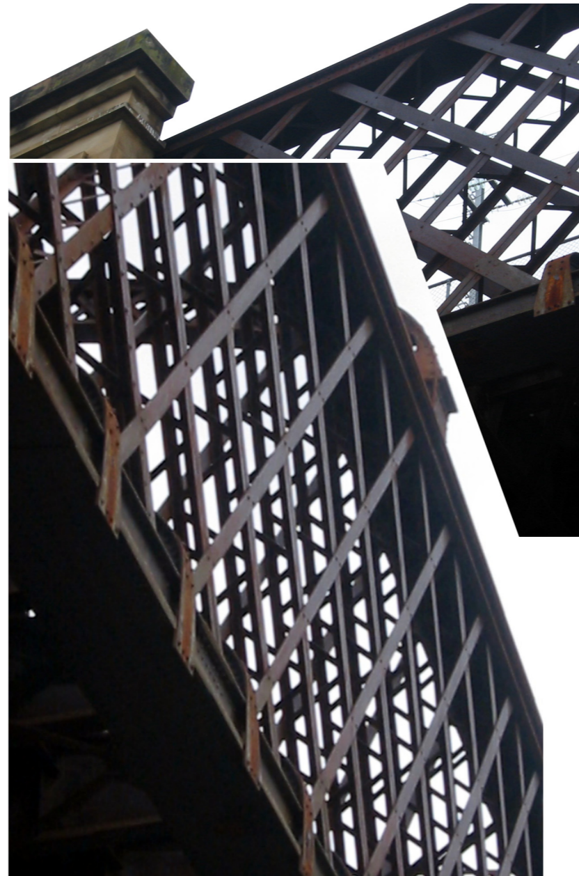
details of the nearby John Whitton Bridge
